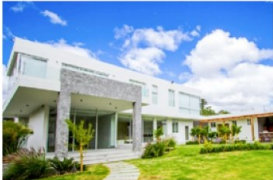
Three-story residence in Vancouver North, Canada
